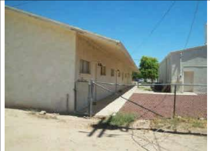
Photo 36: Rear exterior view south end of classroom building.
