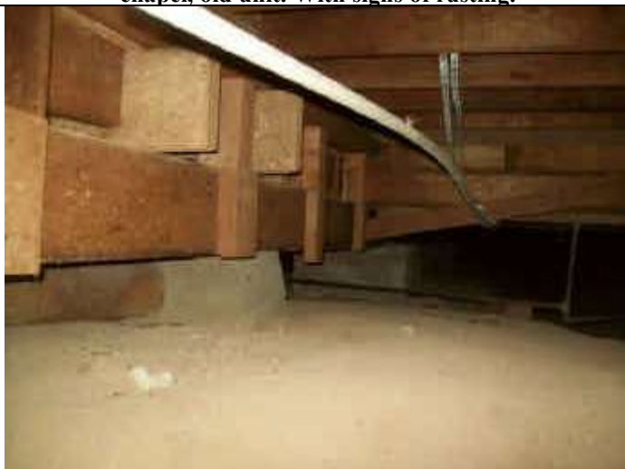
Photo 113: Crawl space view under main chapel area showing wood pier, post and beam supports.
