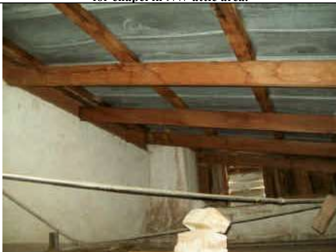
Photo 89: Attic view over chapel area showing substrate and metal roof installation.
