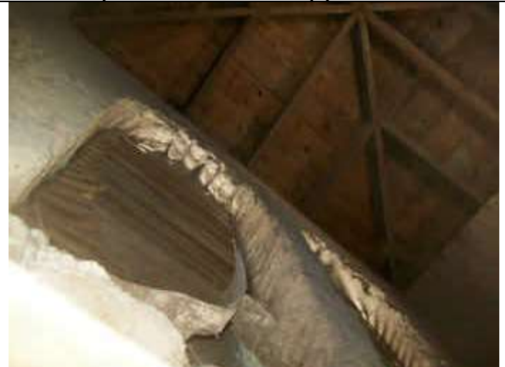
Photo 72: View in attic area or bell tower of chapel where old bell installed.
