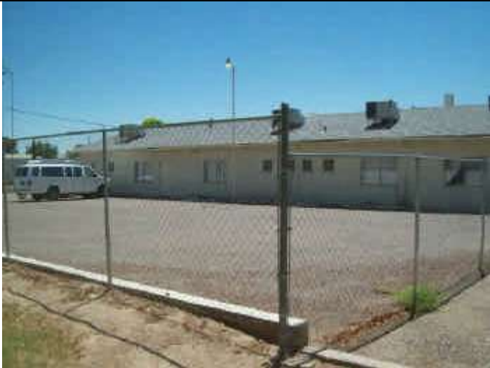
Photo 7: North exterior view of classroom and parking area looking SE.
