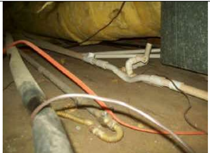
Photo 96: Older gas line not in use by HVAC units in chapel.
