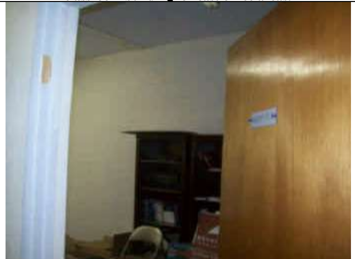
Photo 48: Study or library in classroom building at NE corner.
