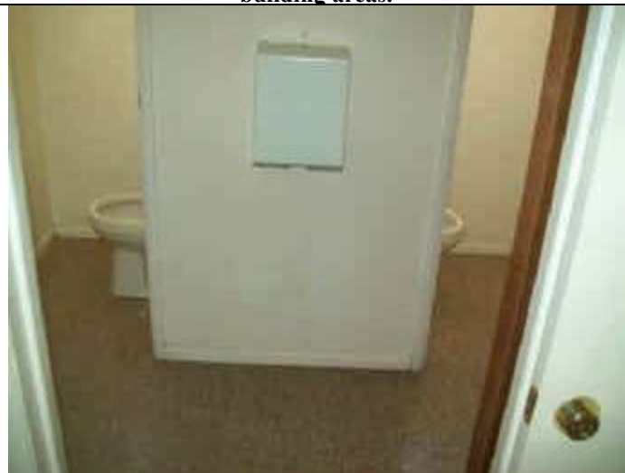
Photo 57: Common restrooms for kitchen and social hall areas.
