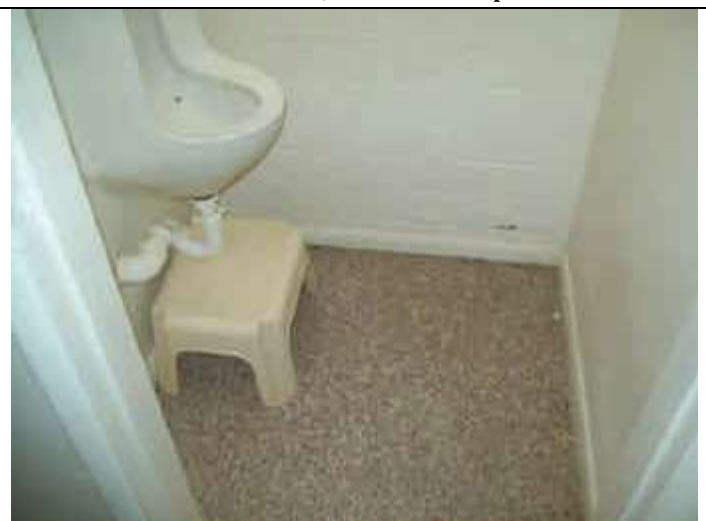
Photo 60: Urinal view in men's restroom in kitchen area.
