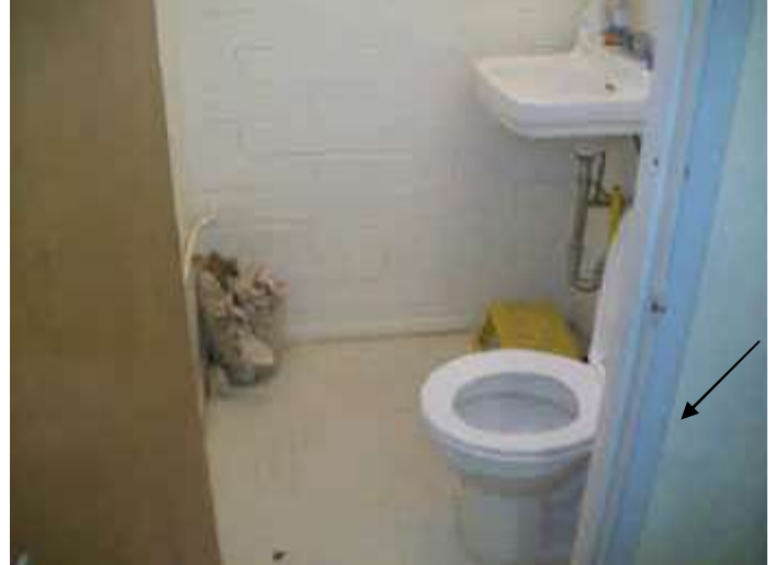
Photo 46: Common hallway restroom in hallway of classroom building for east office areas.
