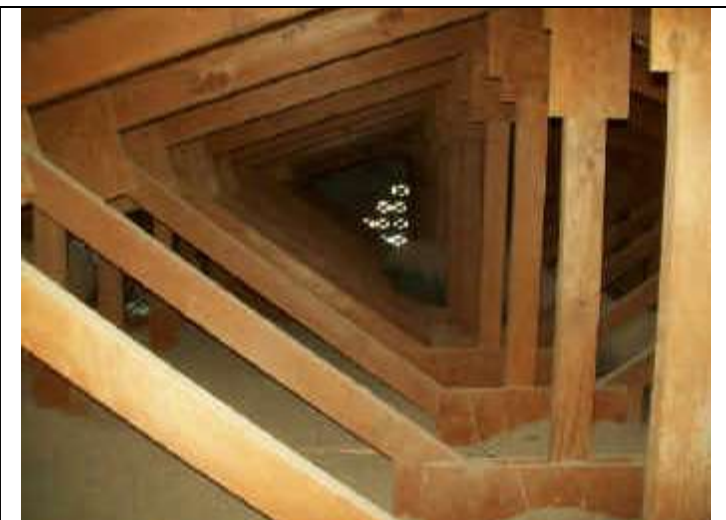
Photo 38: Attic view over classroom building showing site-built truss and sheathing construction.
