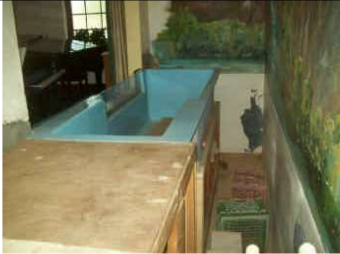
Photo 79: Baptismal bath tub view in chapel by alter area.
