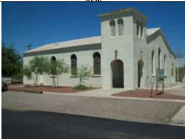
Photo 3: South exterior view of chapel.
