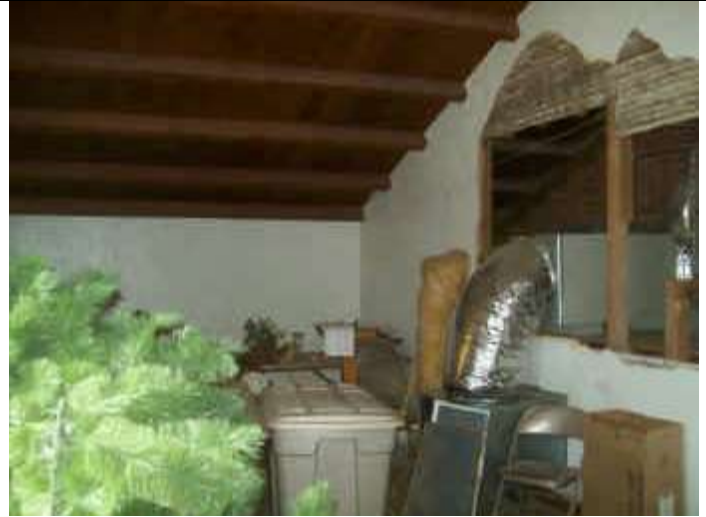
Photo 92: Rear interior storage area of chapel and access to HVAC air handler installations.
