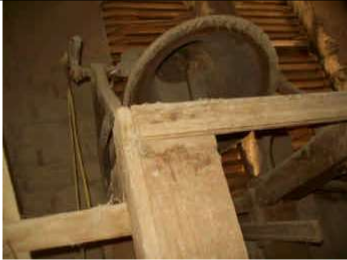
Photo 73: View in attic area or bell tower of chapel where old bell installed.
