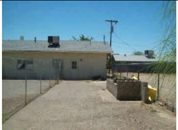
Photo 8: North exterior rear end view of classroom building looking south.
