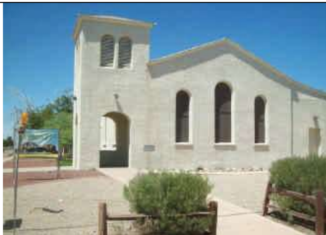
Photo 1: Front exterior view south end of chapel looking west.
