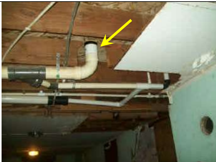
Photo 105: Floor joists cut to install plumbing along top ceiling area of basement.
