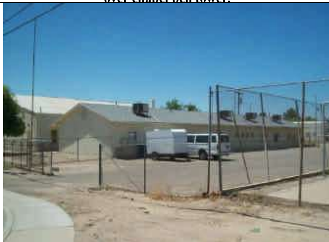
Photo 4: North exterior view of classroom building and parking area.
