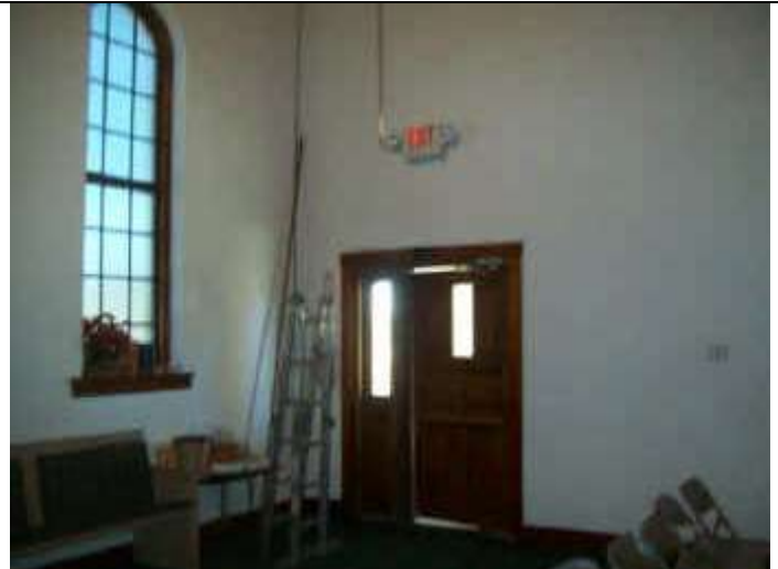
Photo 76: Entry view to chapel area looking south.
