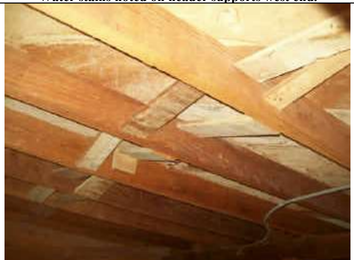
Photo 114: Crawl space view under main chapel area showing wood substrate and supports.
