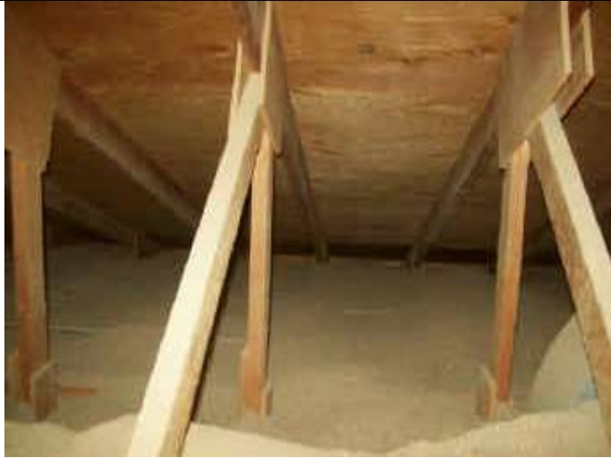
Photo 39: Attic view over classroom building showing wood truss, sheathing and insulation installations.
