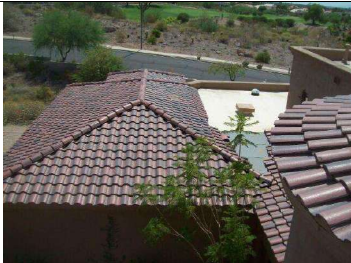
Photo 33: Main house concrete tile and rubber membrane roof surface view, typical.
