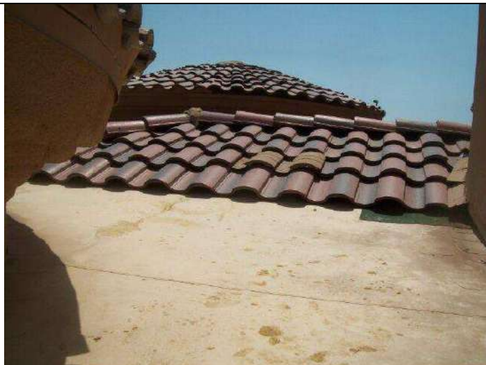
Photo 21: Main house concrete tile and rubber membrane roof surfaces view, typical.
