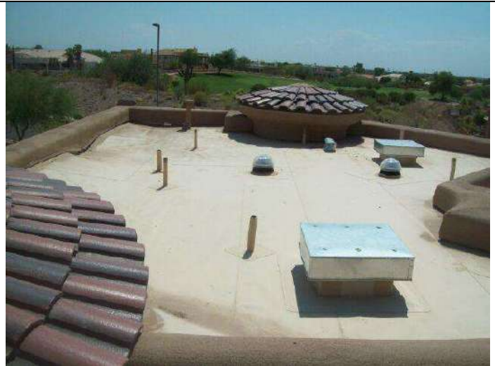
Photo 38: Main house concrete tile and rubber membrane roof surface view, typical.
