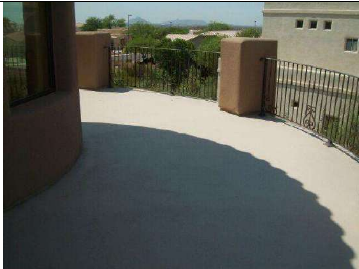
Photo 31: Upper level deck surface view, typical.
