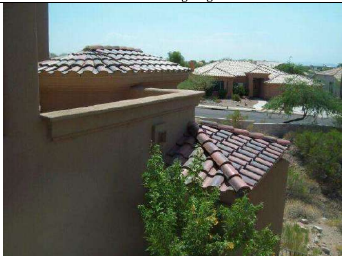
Photo 29: Main house concrete tile roof surface view west slope and typical.
