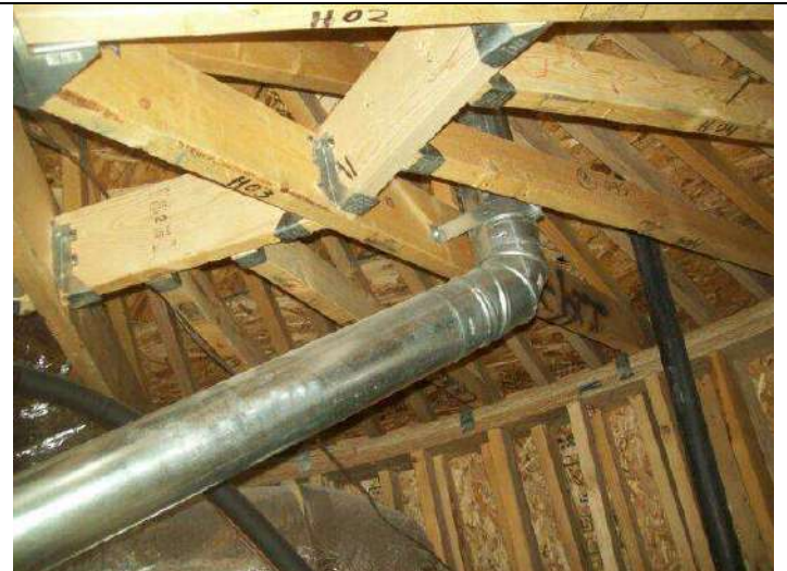
Photo 28: Attic view showing wood truss and sheathing installations.
