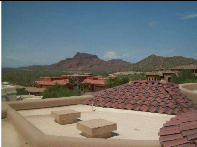
Photo 39: Main house concrete tile and rubber membrane roof surface view, typical & view of north mountain range.
