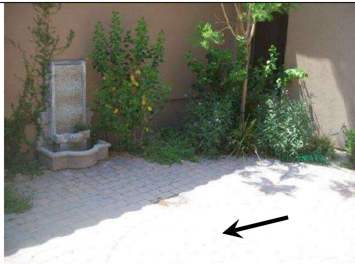
Photo 14: Drain line in front courtyard area.
