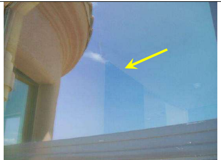
Photo 30: Scratching on surface of west exterior window upper level.
