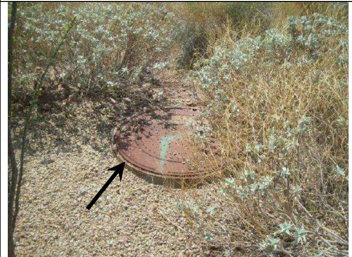
Photo 10: City sewer manhole at SE corner of property.
